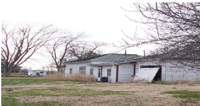
Photo of the Palmer property prior to demolition
